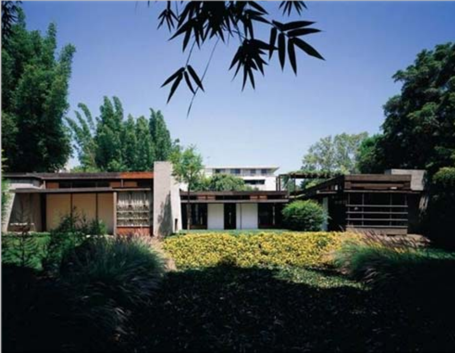
Rudolph M. Schindler, Los Angeles Kings Road House, 1921–1922 Fitzpatrick-Leland House, 1936 Pearl M. Mackey Apartments, 1939
